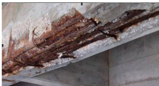
FIG.5.1.6B-corrosion of reinforcement
